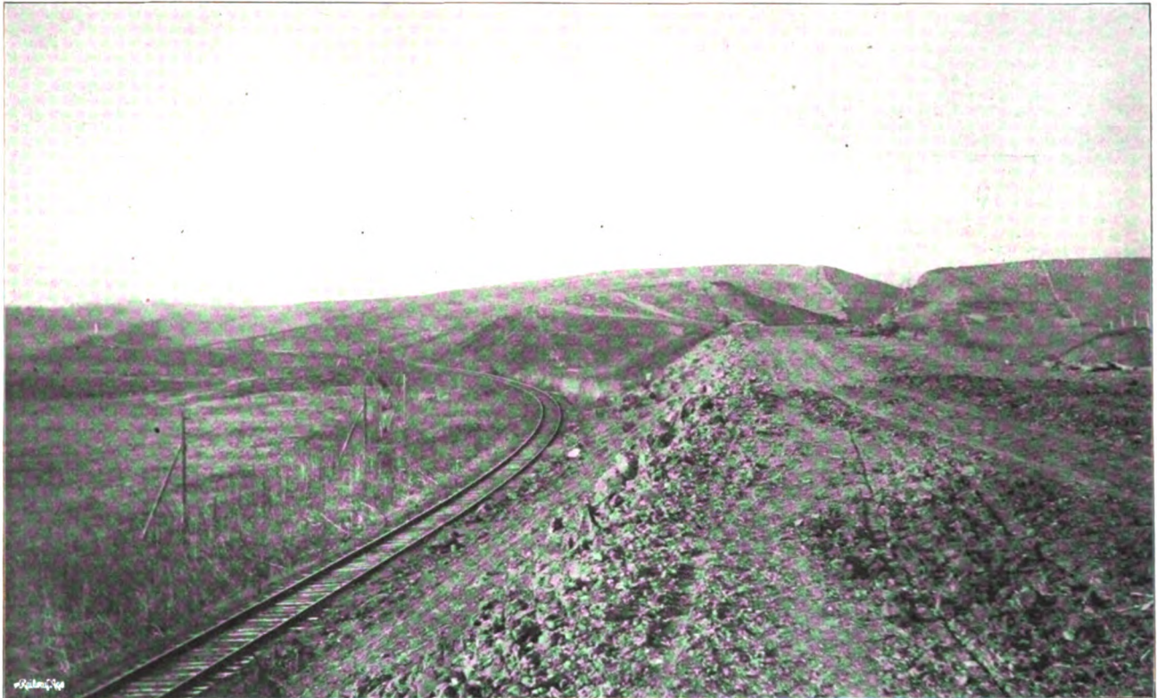
C. B. & Q. RELOCATION—LOOKING WEST ALONG THE NODAWAY FILL TOWARDS THE VILLISCA CUT.
