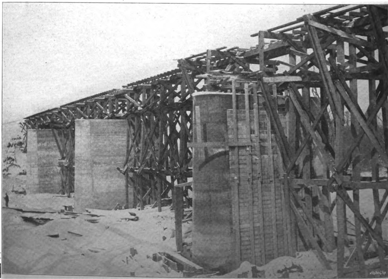
C. B. &amp; Q. RELOCATION—CONCRETE PIERS AND TEMPORARY TRETTLE AT WEST NODAWAY RIVER.
