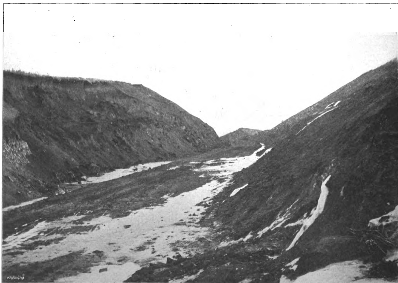
C. B. & Q. RELOCATION—85-FOOT VILLISCA CUT, LOOKING EAST.
