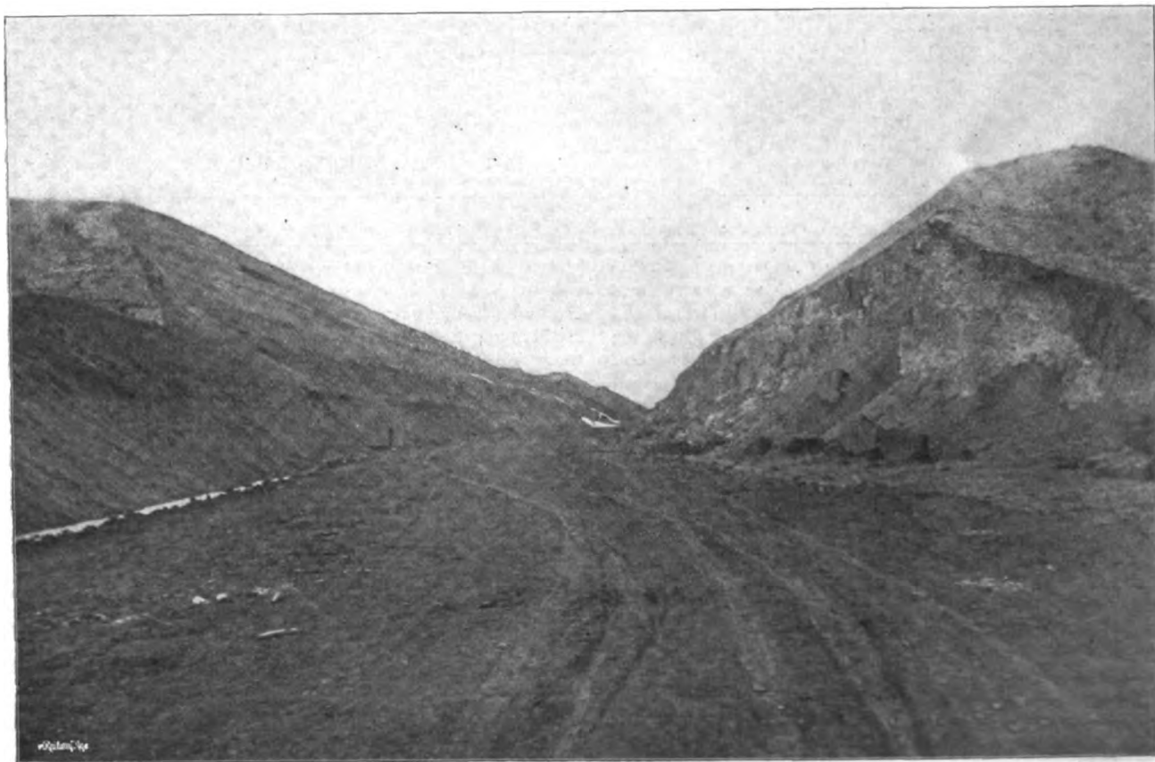
C. B. & Q. RELOCATION—85-FOOT VILLISCA CUT, LOOKING WEST.
